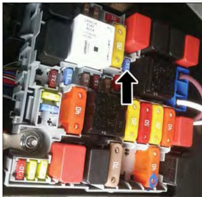
Power Outlet Fuse Location
