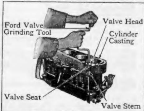
Method of grinding valve. (Cut No. 5)
