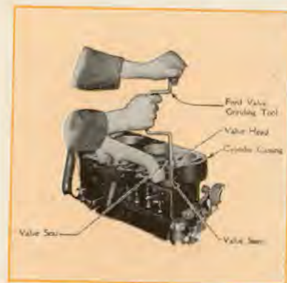
Method of grinding valve. (Cut No. 6)
